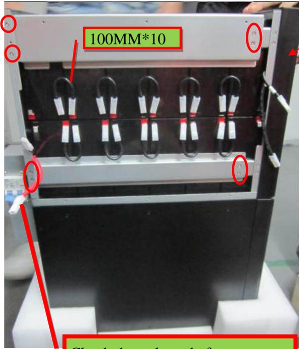
Screw up the guardrail like the picture on the left;
