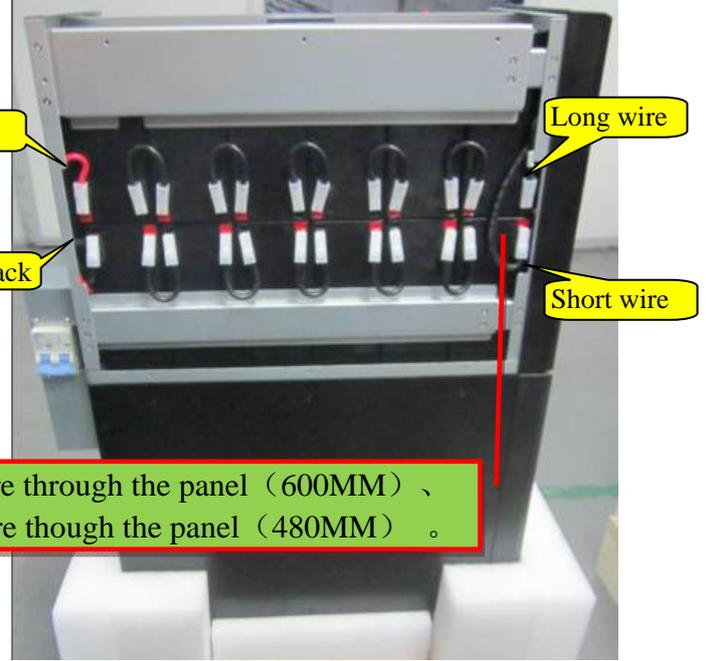
Long wire through the panel (600MM) , Short wire though the panel (480MM) 。
